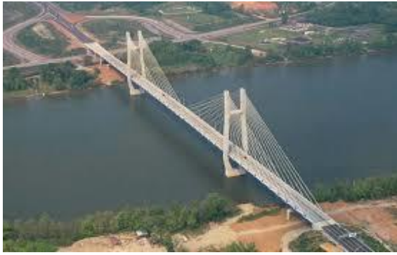
Fig. 1. William H. Harsha Bridge [6].
