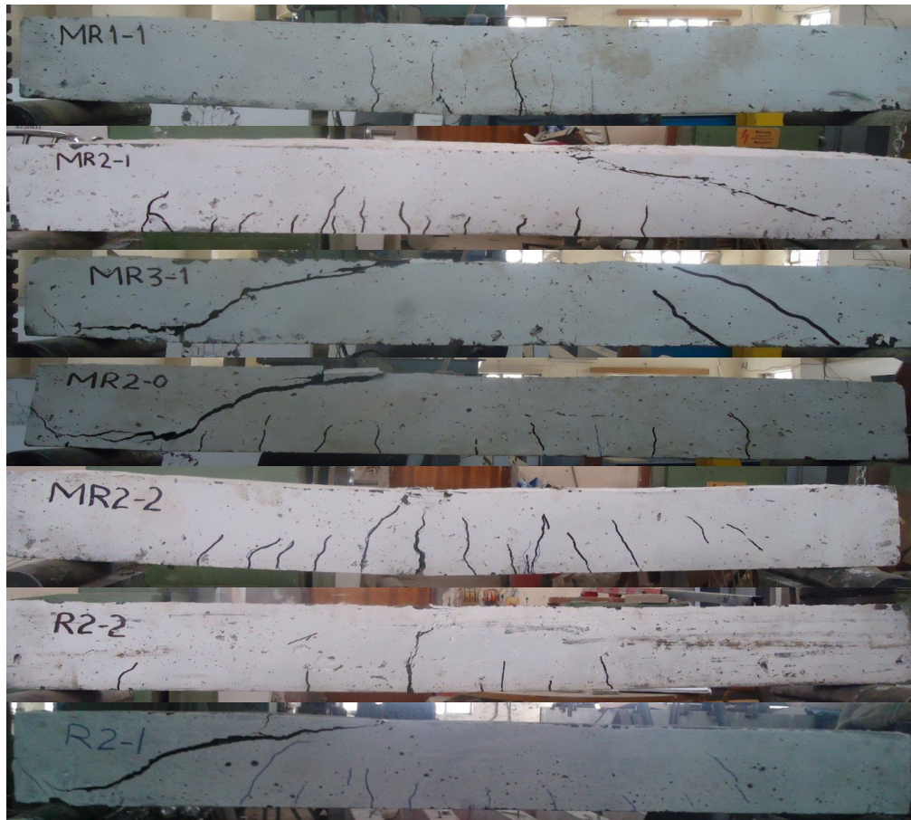
Figure 12. Crack patterns of the tested beams
