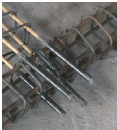
Figure 6. GPRF bars with mechanical couplers before molding
