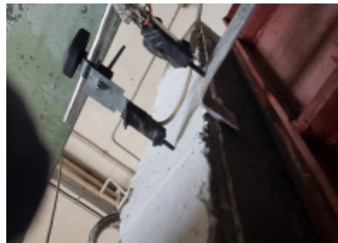
(d) Installation of LVDT on the edge of concrete and steel plate
