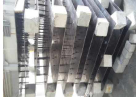
(b) slabs prepared before concreting
