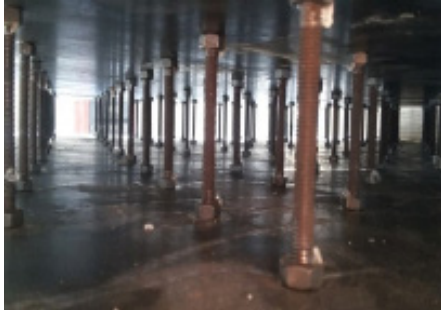
(a) assembling plates and stud bolts
