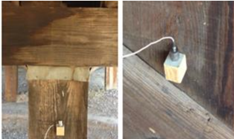
Fig. 7. Accelerometers Mounted on a Pile Side Using Wooden Blocks.
