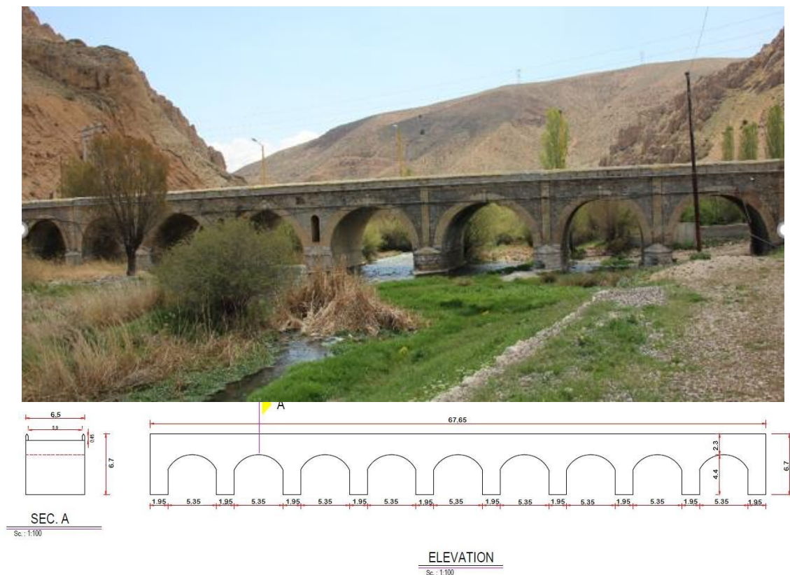
Fig. 6. A view of the Namroud stone bridge and its dimension.
