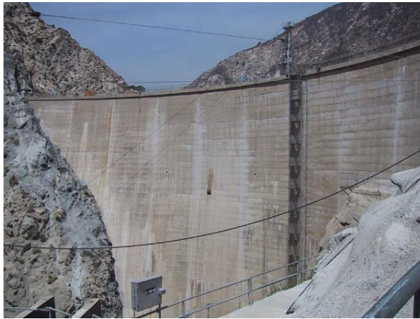
a) View of the right abutment
