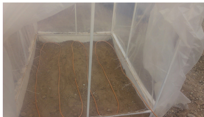
Fig. 3. The cupric tube in the floor of greenhouse
