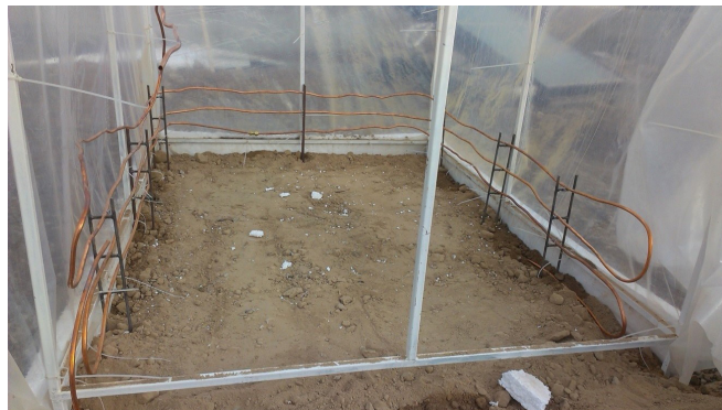
Fig. 4. The cupric tube in the edges of greenhouse
