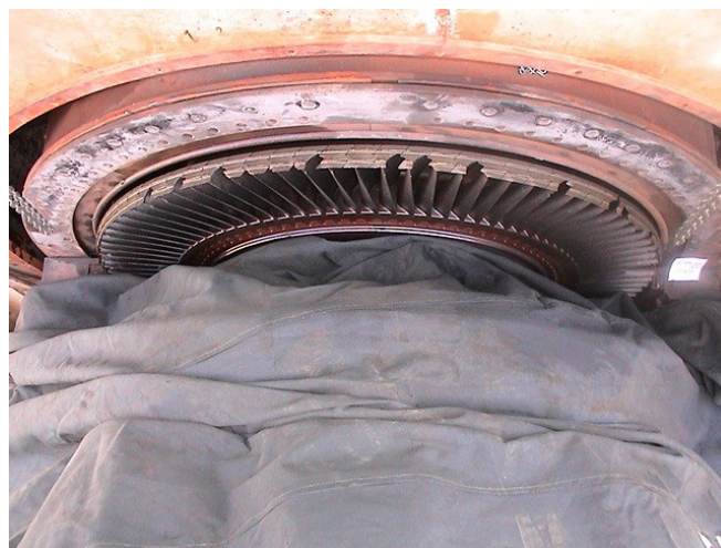
Fig. 1. The general view of the failure in the gas turbine
