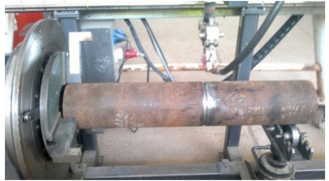
Fig. 6. Welding of pipes
